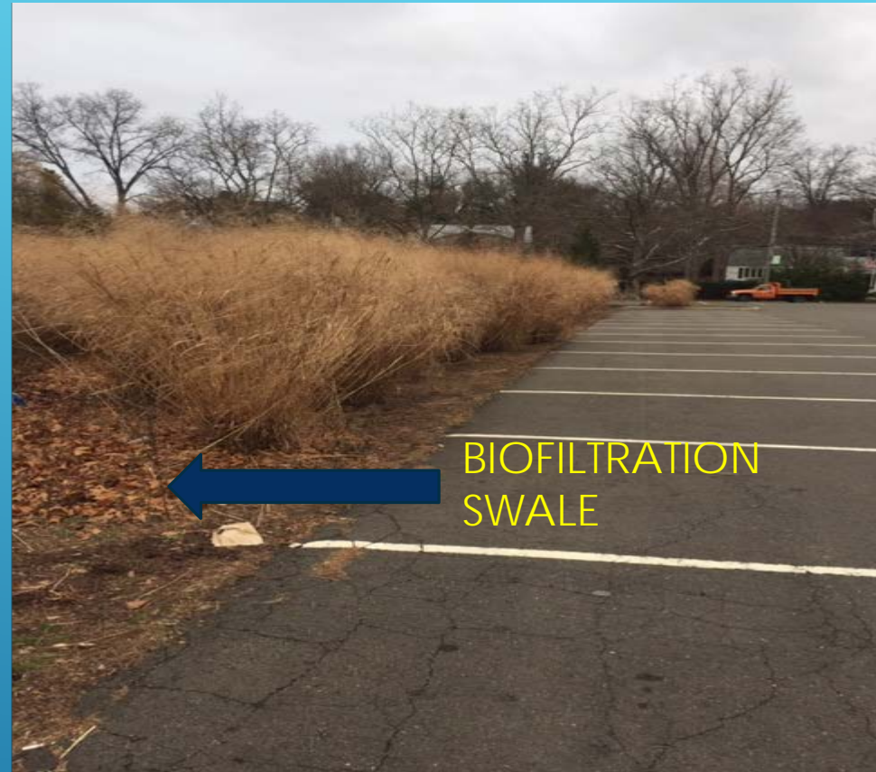
PAR 3 GOLF COURSE- TENNIS CENTER PARKING LOT- SOUTH PINE CREEK ROAD
