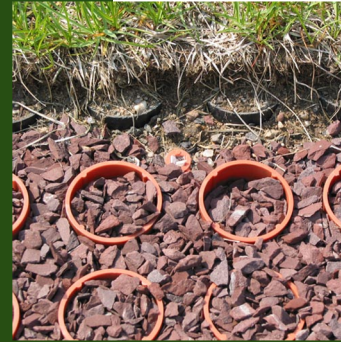
Gravel Grid Pavement
