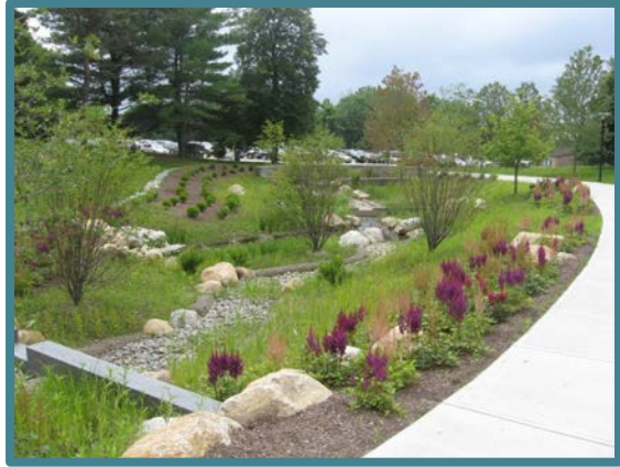
Rain Gardens and Bioretention System
